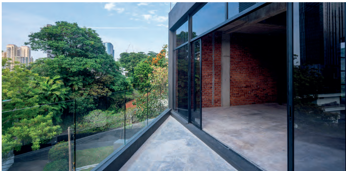
(Facing page) Driving uphill towards Project Conservatory gradually reveals its massive brick façade walls. (Above) Grey-tinted glass sliding doors help keep the interior of the house cool.
