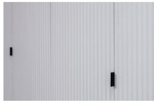
Detail - vertical lines forming a backdrop to the space
